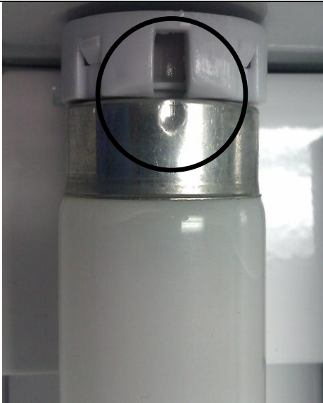
Diagram 1-T8 lamp seating
