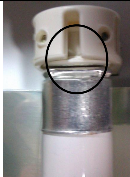
Diagram 2-T5 lamp seating
