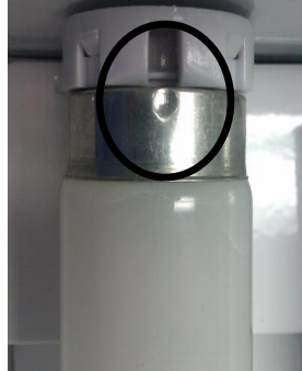
Diagram 1-T8 lamp seating
