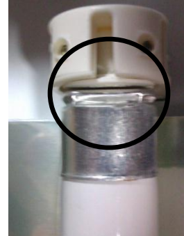
Diagram 2-T5 lamp seating
