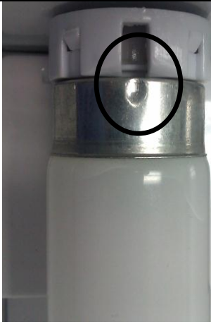
Diagram 1-T8 lamp seating
