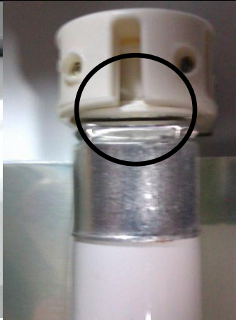
Diagram 2-T5 lamp seating
